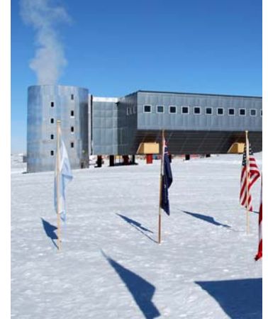
Amundsen-Scott South Pole Station Image Credit: Dwight Bohnet, National Science Foundation
